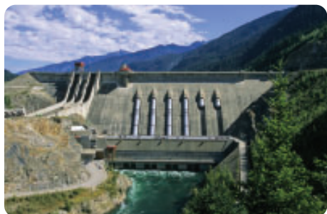
Figure 2 Revelstoke Hydroelectric Dam in Revelstoke, B.C.
