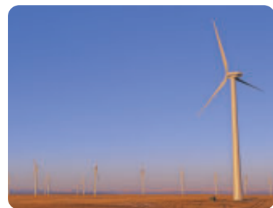
Figure 4 Under typical wind conditions, a 2 MW wind turbine can supply more than 500 homes with electricity.
