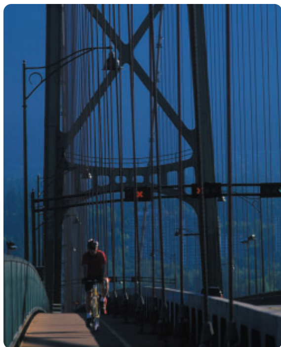
Figure 4 The ductility of some metals and the development of technology that can draw steel into wires make suspension bridges, like the Lions Gate Bridge in Vancouver, possible.
