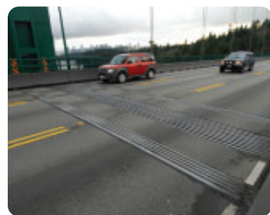
Figure 3 Expansion joints in Lions Gate Bridge, Vancouver
