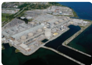
Figure 7 The Pickering Nuclear Plant in Ontario is one of the world's largest nuclear generating facilities.
