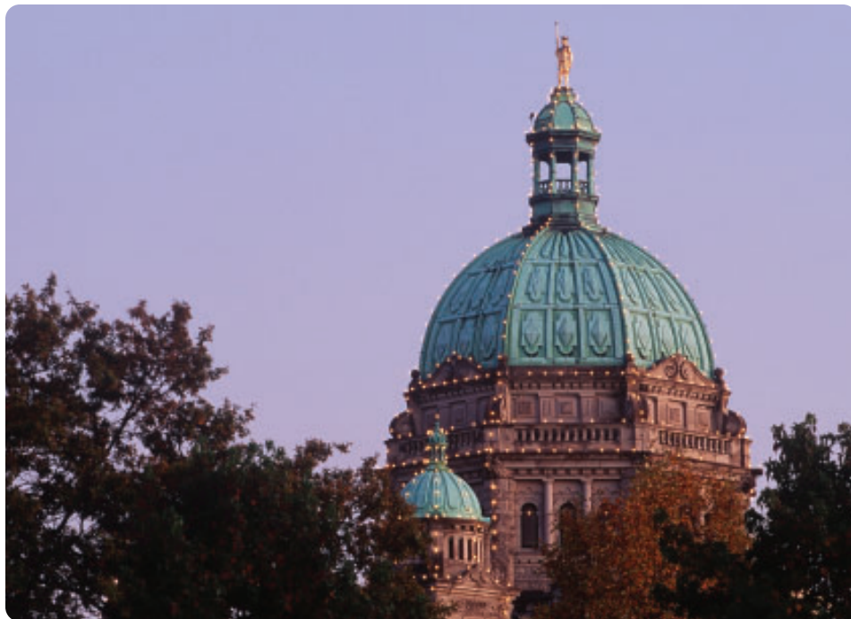
Figure 2 The Legislative Building in Victoria, B.C. The blue-green colour of the copper roof is due to copper(II) ions that form as the copper metal reacts with the atmosphere.
