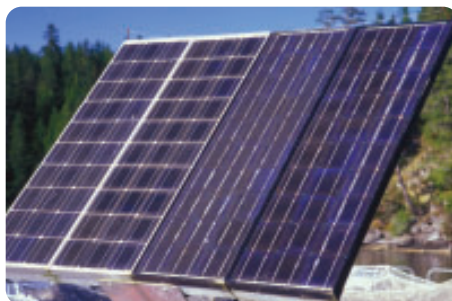
Figure 3 Panels of photovoltaic cells
